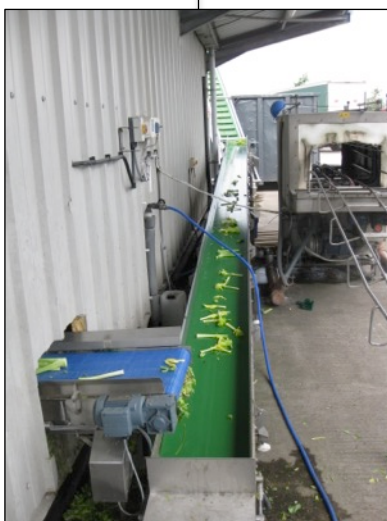
Waste handling system depositing all product waste in skip outside
