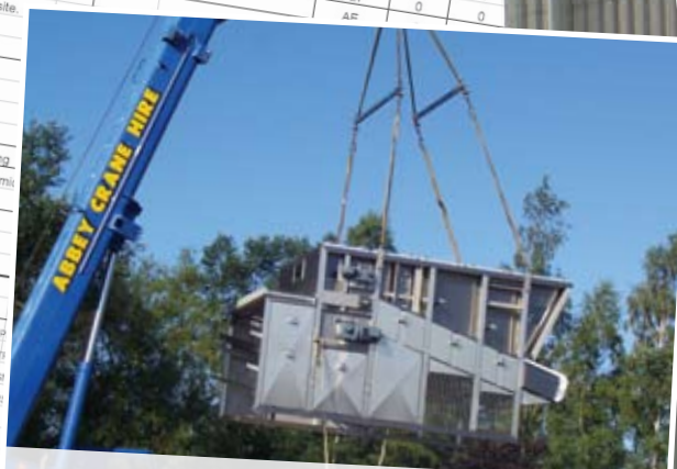
APRON FEEDER BEING LOADED
