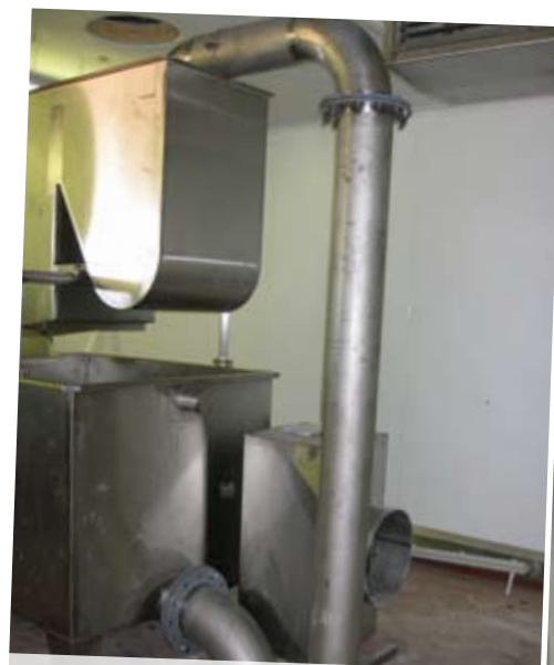
PIPE WORK FOR PUMPING SYSTEMS INSTALLATION
